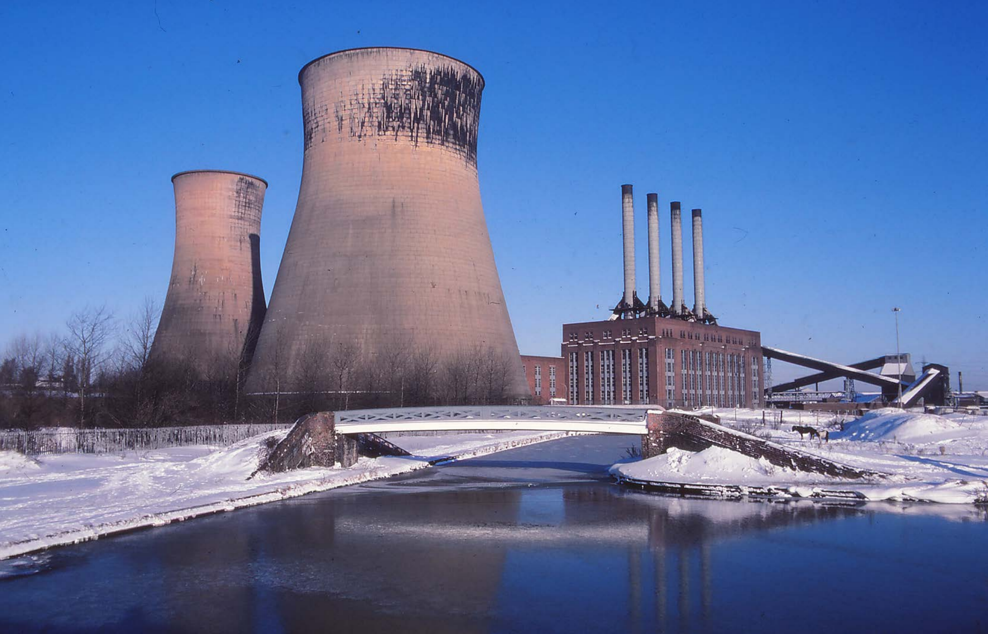
Ocker Hill Power Station, Tipton, 1985; photograph by Keith Hodgkins.
